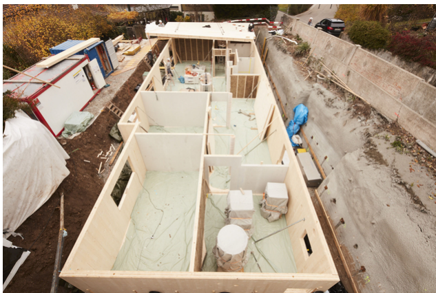
Basement during the construction phase
