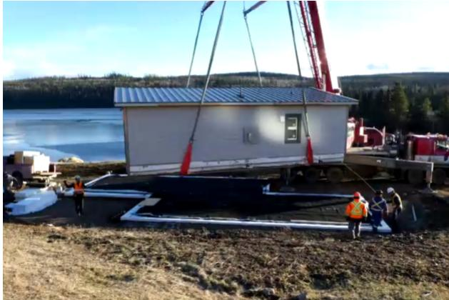
In British Columbia in western Canada, the first innovative residential building with a wooden floor slab has been built. The house impresses with its sustainable construction method, which starts with a wooden floor slab right from the foundation, and is a convincing passive house standard in use.
