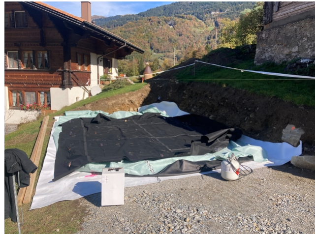
Waterproofing and moisture monitoring is ready
