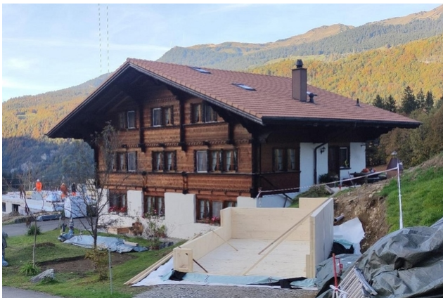
Cross laminated timber boards are grouted
