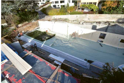
CLT cross-laminated timber panels are used to build the walls.
