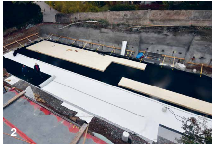
A non-woven fabric is used to safeguard the waterproofing and the integrated full-surface moisture monitoring.
