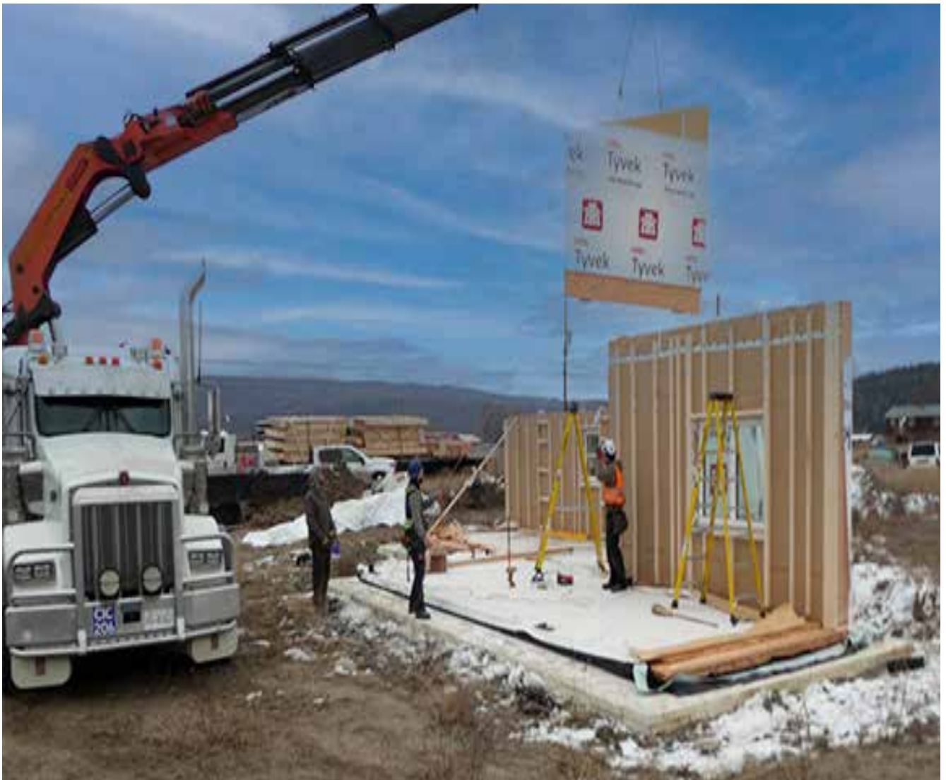
Above this, the timber construction company is installing the subsequent parts of the timber building.
