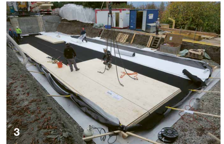
The cross-laminated timber floor slab is laid on the waterproofing and the full-surface moisture monitoring system.
