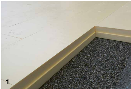
A layer of chippings is used to lay thick insulation boards.
