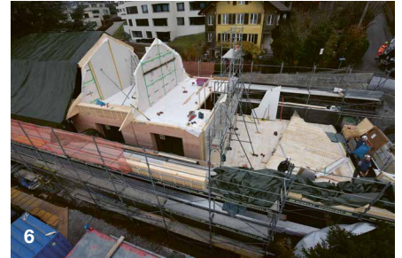
Above this, the timber construction company is installing the subsequent parts of the timber building.
