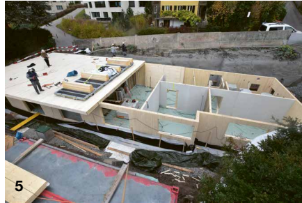
CLT cross-laminated timber panels serve as a load distribution slab.
