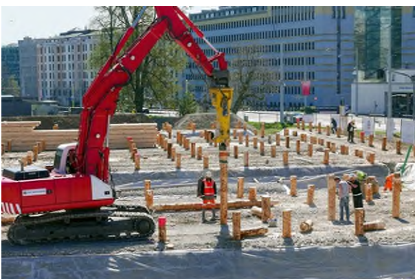
Figure 2. Opera des Nations Geneva, installing the spruce piles, Source [6]
