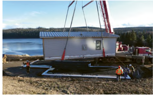
Figure 11. Modular house constructed on a timber slab-on-grade foundation in Canada. Source: www.timbase.com
