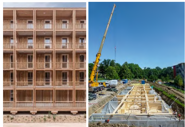
Figure 3. A five-storey apartment building (left) has been built on wooden piles and the construction site of the building (right) [7]
