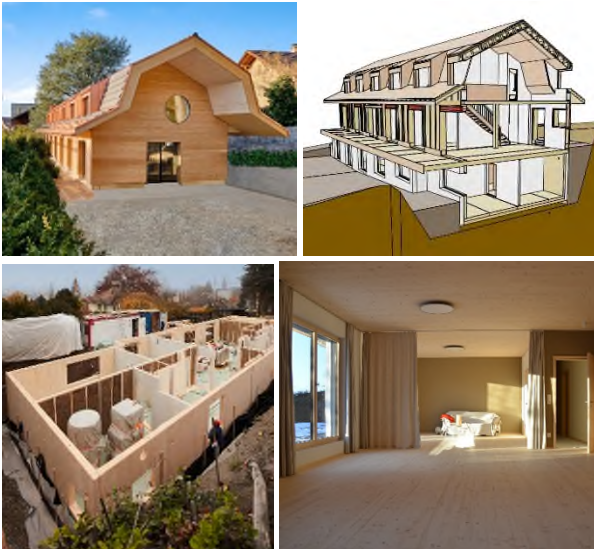
Figure 9. Apartment building in Thun: outside view, visualisation of column and panel construction with TS3, timber basement under construction and interior view of the finished basement (clockwise). Source: www.timbase.com
